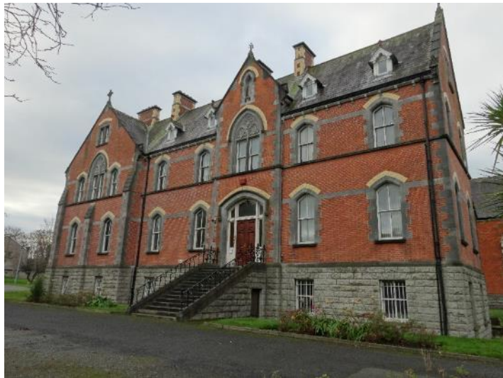
East-facing entrance elevation of L-plan wing dated 1888 (Structure 1)
