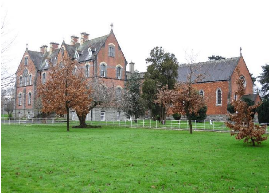
Photo of Structure
