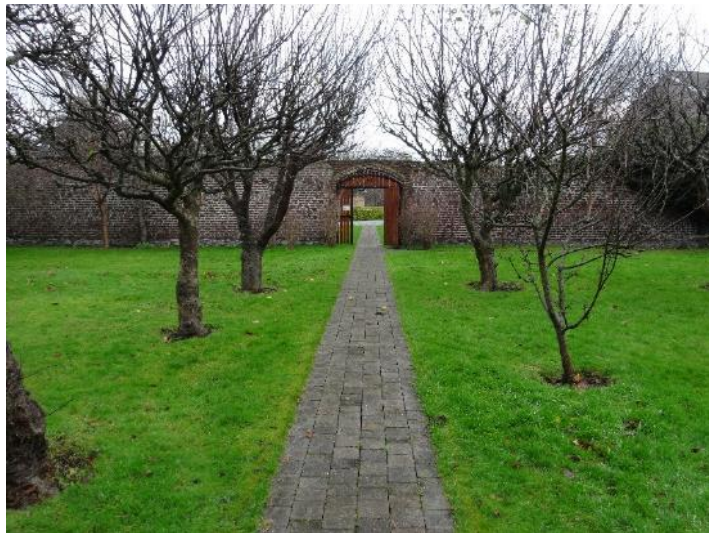
Brick-faced eastern wall with entrance gate to walled orchard. Brick was used to face the wall as it retained the sun's heat and encouraged the growth of espaliered fruit trees ( Structure 7 )
