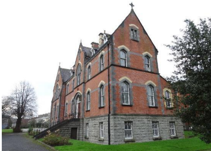
East-facing entrance elevation of L-plan wing dated 1888 (Structure 1)
