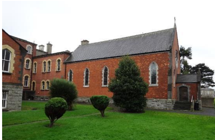
East elevation of the five-bay chapel ( Structure 4 )
